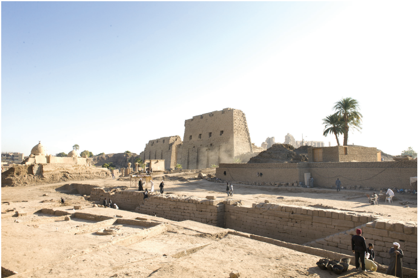
Figure 1 The sand stone embankment.
